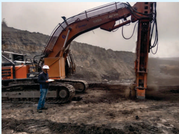
NPC Team studying Drill machine at Sonepur- Bazari OCP, ECL
