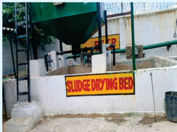
Sludge Dry Bed at M/s. ATO Exim's Pvt. Ltd., Unnao
